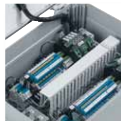
The control box terminals, valve wire sets, and motor contactors are all sealed, labeled, and prewired
